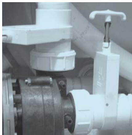
Slice Valve and Pump Union
